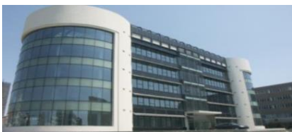
Dalian Rongke Power Co. Ltd. Dalian, China
